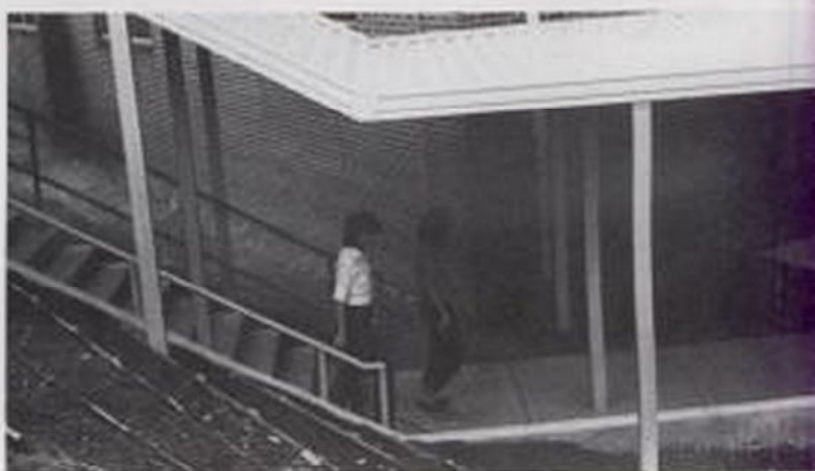
A canopy was built over the walkway between the vocational building and the main building. Here, Terri Hanna and Carolyn McKinney, sophomores, enjoy the fact that they won't get wet when it rains. Top, the band members perform on Halloween night.
